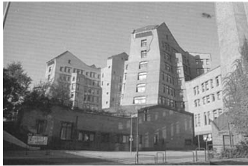
Figure 2.21 NMB Bank Headquarters, Amsterdam
