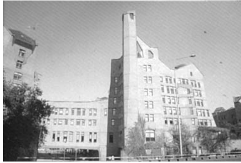
Figure 2.20 NMB Bank Headquarters, Amsterdam
